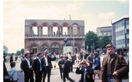
May 1969 - Demolition of the Exchange
